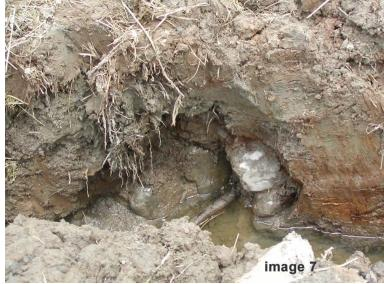
These rocks were unseen underneath where the head of the present pond was developed. All agreed, the remedy was to cut through the head of the big pond and remove these rocks and then rebuild the head (see image 8).
