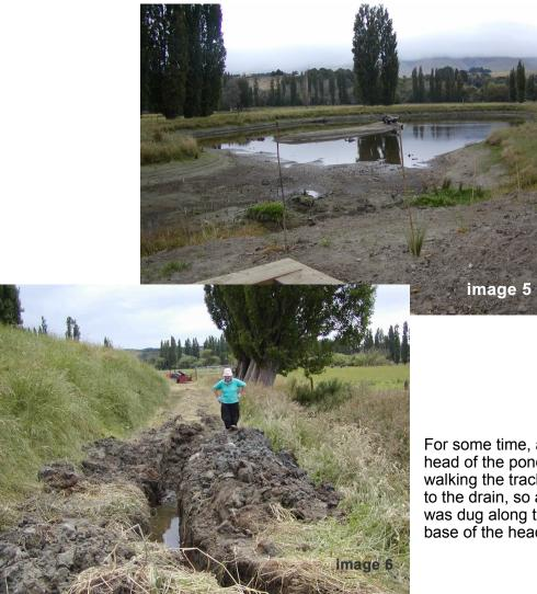
For some time, a wet patch behind the head of the pond was apparent when walking the track behind the head next to the drain, so an exploratory ditch was dug along the pond below the base of the head (see image 6).
